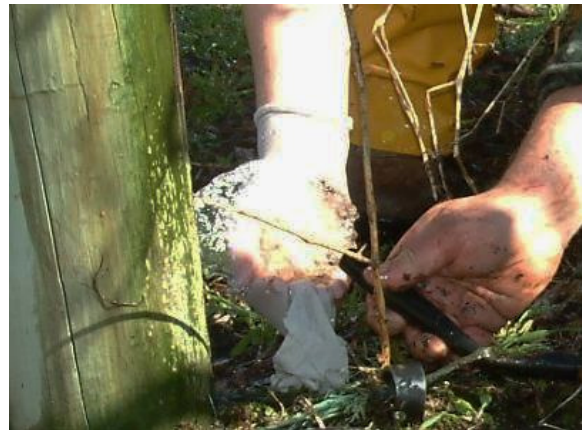
Flushing laterals can help with finding the cause of blockages
