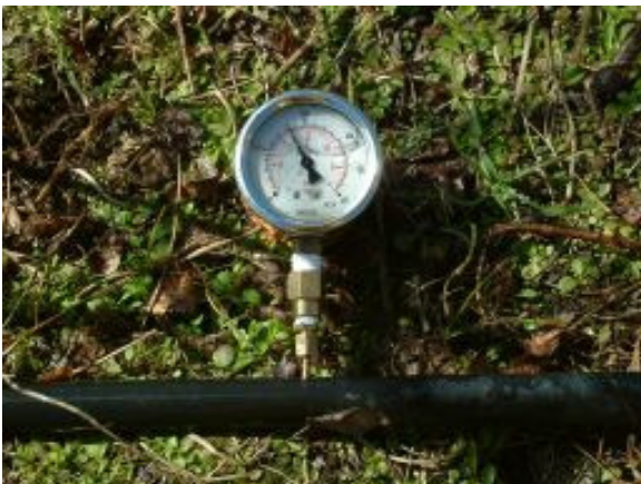
Testing pressure in the laterals
