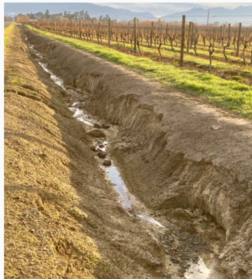
Erosion and sedimentation in a sprayed-out drain
